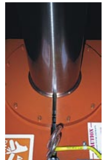
Jaws grip plunger when activated to safely stop elevator.
